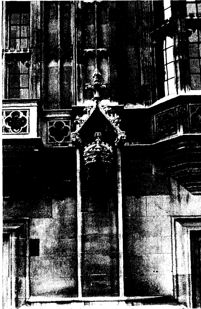
2.1 A.W. Pugin, The Palace of Westminster (from 1845): details of stonework.
