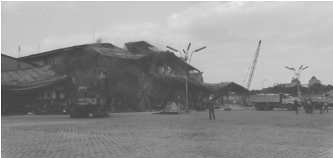
Demolition of cattle market shed, La Villette, Paris, September 1980
