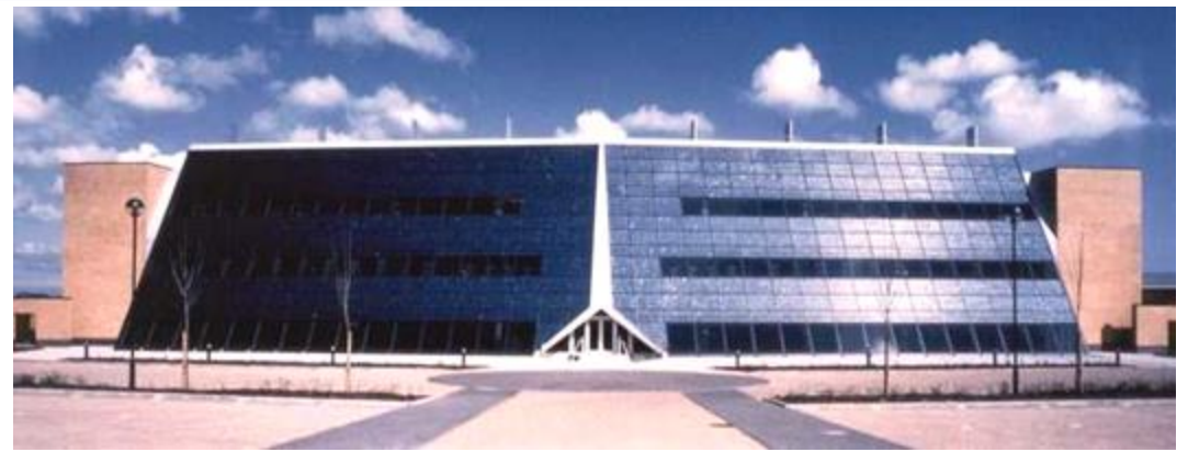
Doxford Int. PLC office, USA: First commercial building with building integrated PV system
